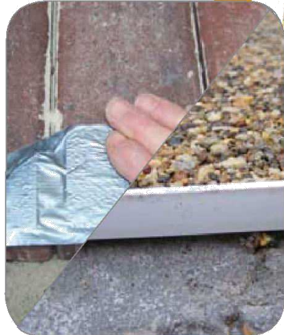
Masking-off with peelable tape & end-stop beading
