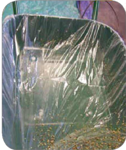
Pour mix into polythene lined wheelbarrow
