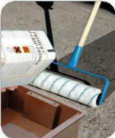
Use Primer C on absorbent surfaces
