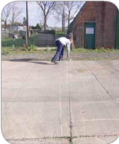
Concrete slab joints
