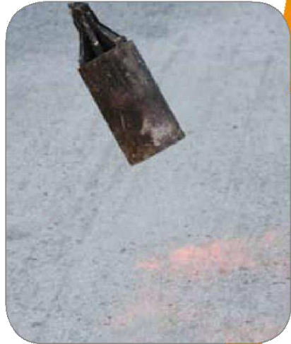
Drying with a hot air lance
