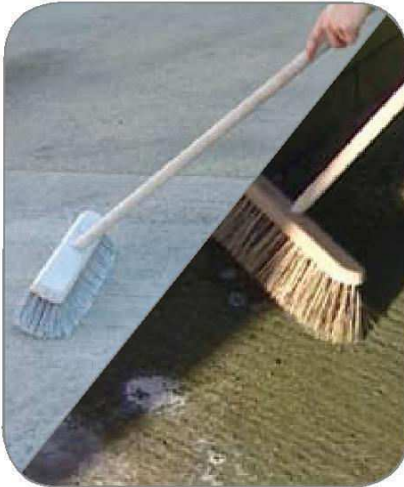
Brushing the surface and removing contamination
